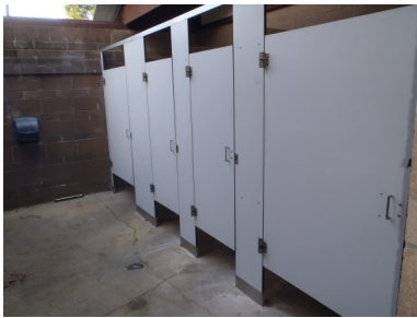
Measure "L" funded: new stall doors in the swimming pool bathrooms.
